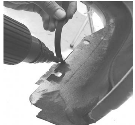
Here the hot air welder is shown in position to start a repair of a torn mounting hole with the R13 PP strip.
